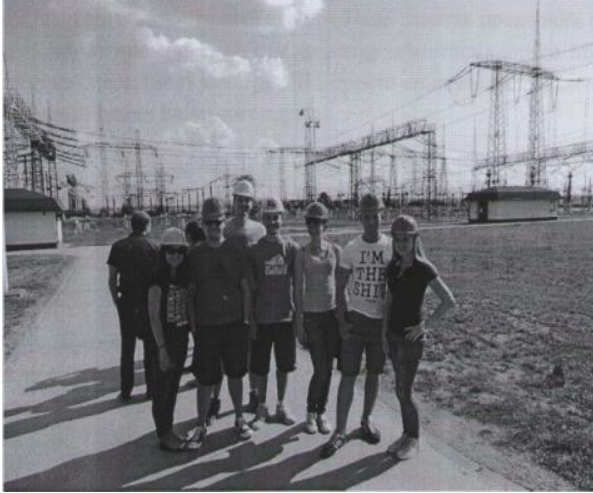
At the ENERCON plant. Photo from the personal archives of A. Yesaulenko
